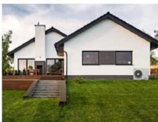
Air Source Heating
